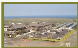
West Hawai'i Civic Center 1st Feed-in Tariff Project
